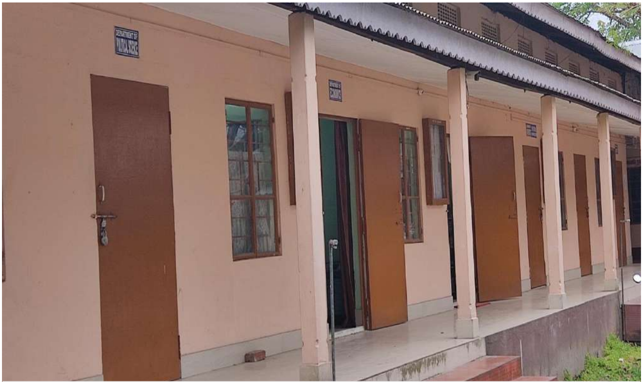
DEPARTMENTAL BLOCK (PARTIAL VIEW)
