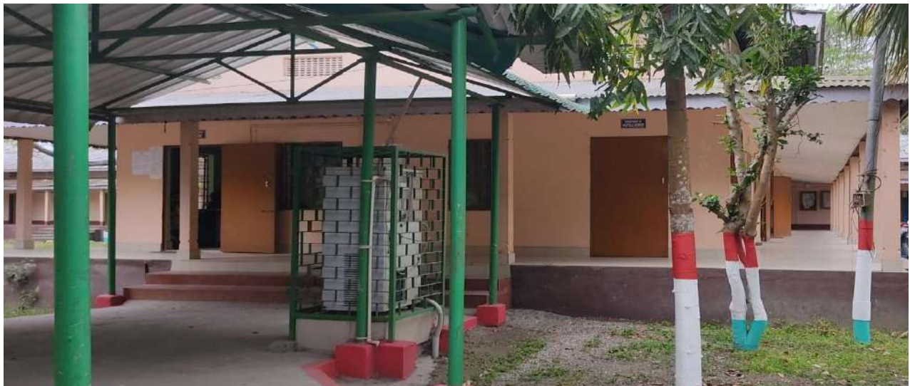
DEPARTMENTAL BLOCK (PARTIAL VIEW)
